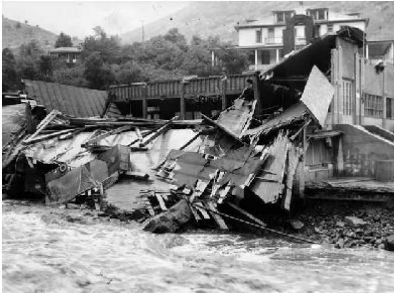
Figure 4-18 Damage to Eldorado Springs Resort, 1938 Flood
